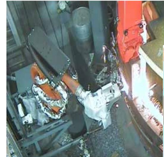
Thermal Cutting Sequence of the Reactor Vessel in the Core Zone
